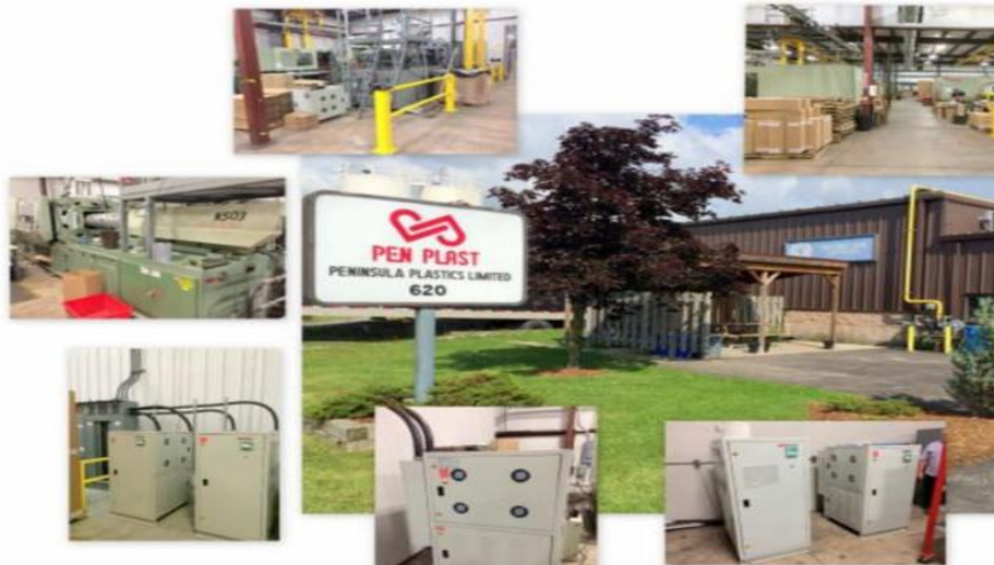
Figure 6. Site and installed project components.
